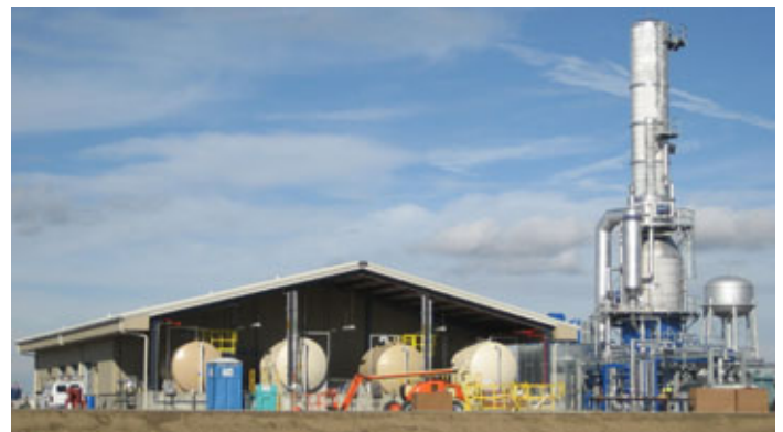
Tracy RO & ZLD Project, brine concentrator on right
